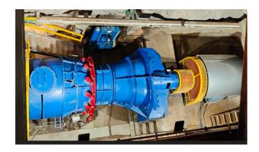
A notable aspect of the turbine is not only its use of diverted canal water to generate electricity—driving the turbine located in the old Fàbrica Vella building (a former textile colony that harnessed water power for energy)—but also the fact that it operates while continuously respecting the ecological flow of the Llobregat River as mandated by regulators.
